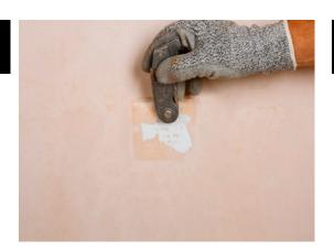
Locate and tap lightly with the head of a screwdriver (or similar) on central area which will loosen the plaster on the face of the bead. Continue until the cut line is visible.
