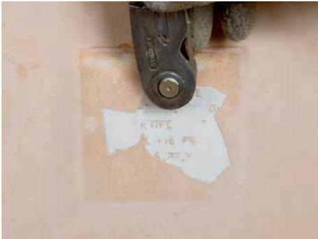
Allow plaster to adequately dry, the bead can be painted over either prior to cut-out or after.
