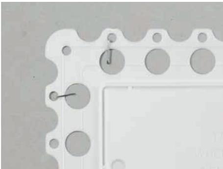
Ensure the bead is attached flush and firmly to the wall.
